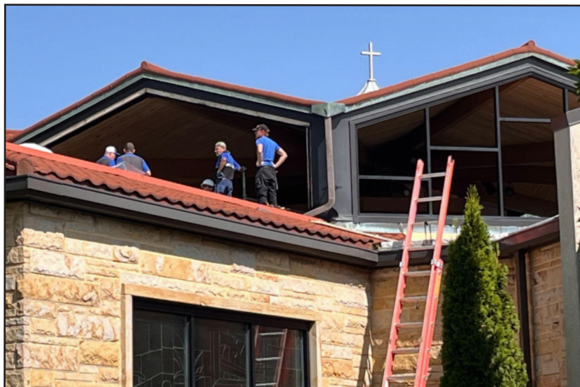
Once the panes were removed, the structure was inspected and necessary repairs were made. The entire panel was removed, but the framework for the window panes was saved and reused.
