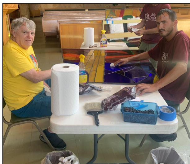
Tom Cullen and crew meticulously cleaning decades of dirt off of the art glass. Not a single pane was cracked or broken.
