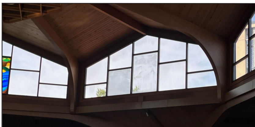
Before removal - glass from the double pane glass had failed, leading to stains and condensation.
