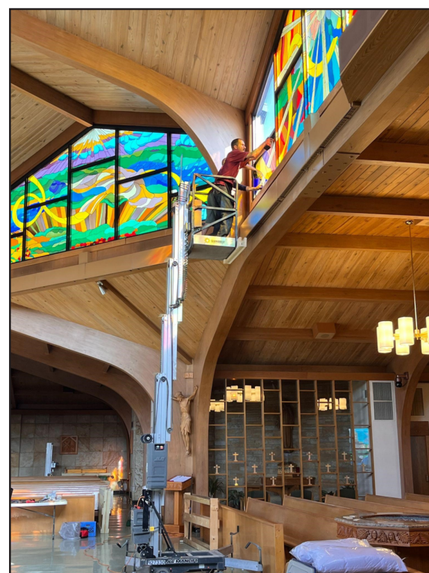
After replacement - the new glass was installed with the repaired structure and care to prevent water damage in the future.
