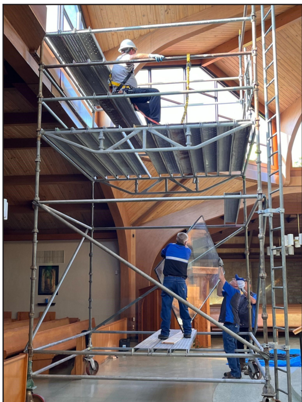
All Service Glass taking down each old pane using the scaffolding.
