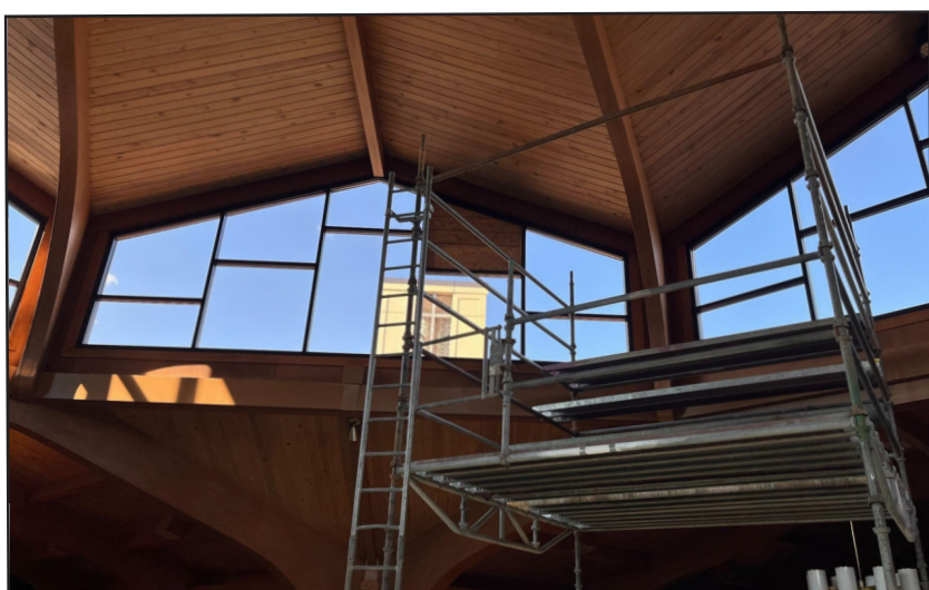
Once the clear panels were replaced and cleaned, the art glass was reinstalled.
