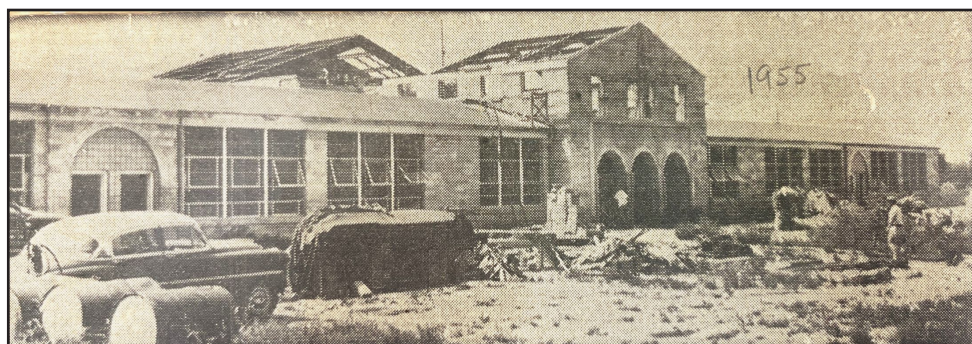
St. Charles School under construction in 1955.
